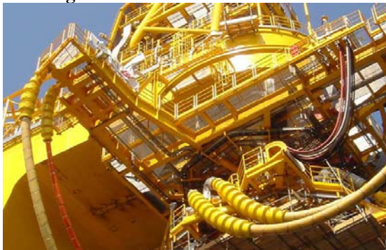
Figure 1. PU Bend Restrictor in Service
